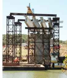
The bulb-tee pier girders were 135' long by 9' to 16' deep along with 185' long by 9' tall drop in girders to make up the 325' span. With the size and weights nearing 250 tons, these beams were delivered to the jobsite from PSI's production and state of the art barge loading facility in Melbourne, KY. The remaining spans were transported to the jobsite by overland truck.
