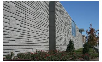
"Precast was selected for the exterior of the arena for economical reasons, and the challenge was to create a precast panel that did not look plain on the tall walls. The solution was a textured liner with a pattern intricately laid out to match each adjacent panel. The result was a unique façade that still complements the surrounding architecture and pays tribute to the region."
